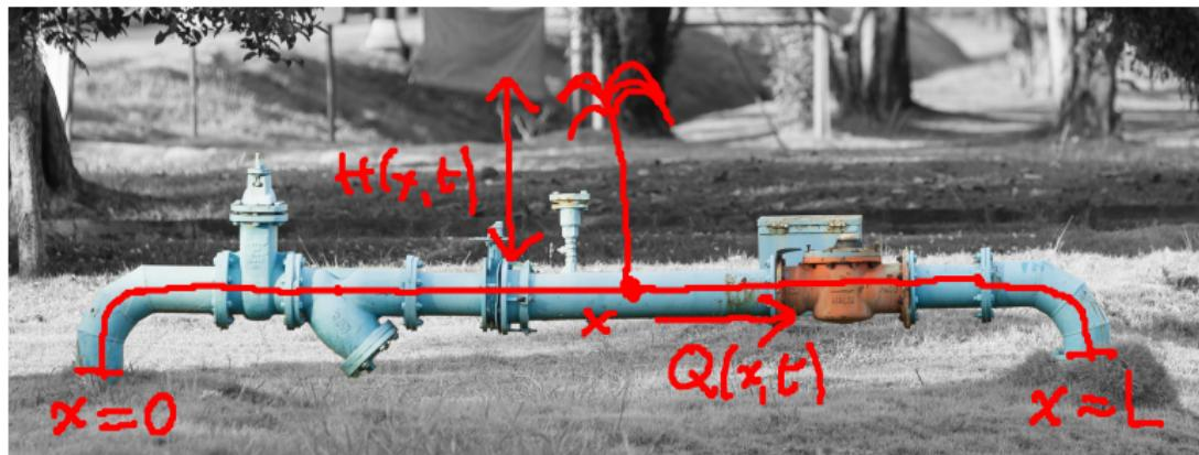
$$\begin{aligned}\partial_t H + \frac{a^2}{gA} \partial Q &= 0, & 0 < x < L, \quad t \in \mathbb{R}, \\ \partial_t Q + gA \partial H &= 0, & 0 < x < L, \quad t \in \mathbb{R}, \\ H = Q &= 0, & 0 < x < L, \quad t \leq 0.\end{aligned}$$
